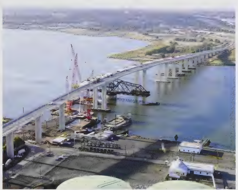
Victory Circle elimination and Victory Bridge replacement project were completed in 2005.
